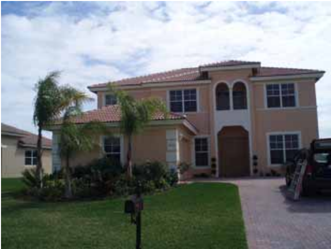
Site photo. The front of the house faces towards the north.
