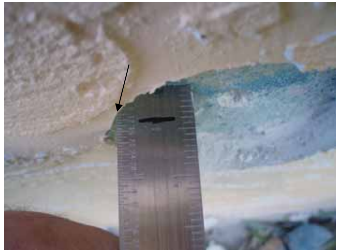
The thickness of the stucco was 3/8 " at this location.
