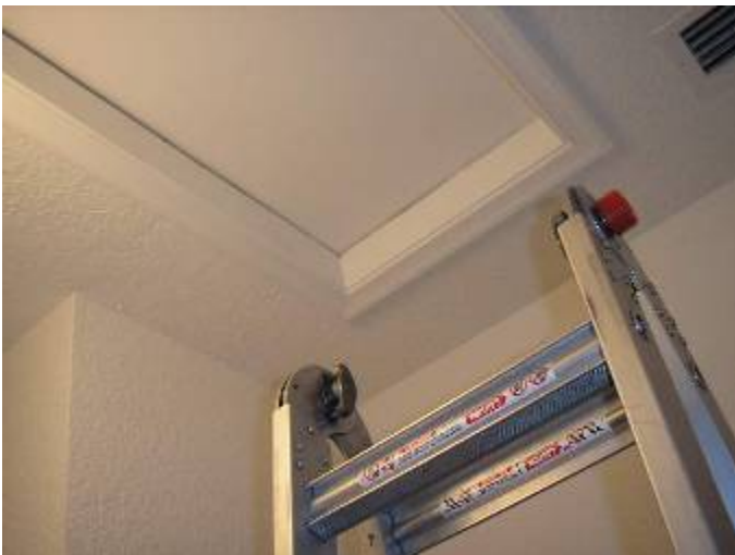
Attic inspection begins.
