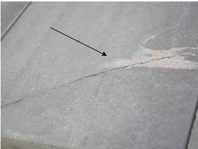
There were broken & incorrectly repaired roof tiles at several locations. The broken roof tiles should be removed & replaced, not "glued" back together.
